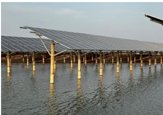
Solar photovoltaic panels rise above an aquaculture farm in Dongying City, Shandong Province, China. The panels, which not only produce enough energy to power 113,000 houses, help cool waters which has helped to boost shrimp and sea cucumber yields by 50%.
